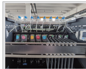
Sub Tank Heating
